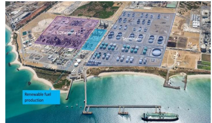
BP's former oil refinery site in Kwinana will host a plant for sustainable aviation fuel as well as a green hydrogen plant.
